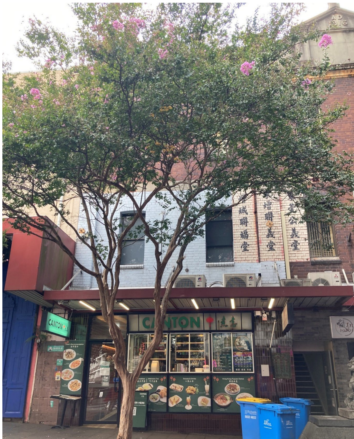
Figure 26. View of 50 Dixon Street. Source: HAA, 2024.
