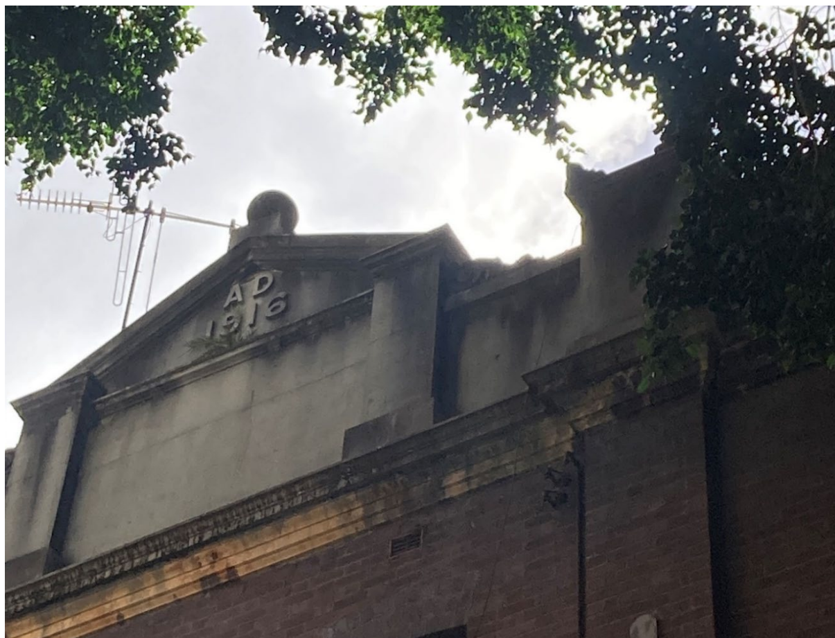
Figure 25. Pediment and architrave detailing on 50-54 Dixon Street. Source: HAA, 2024.
