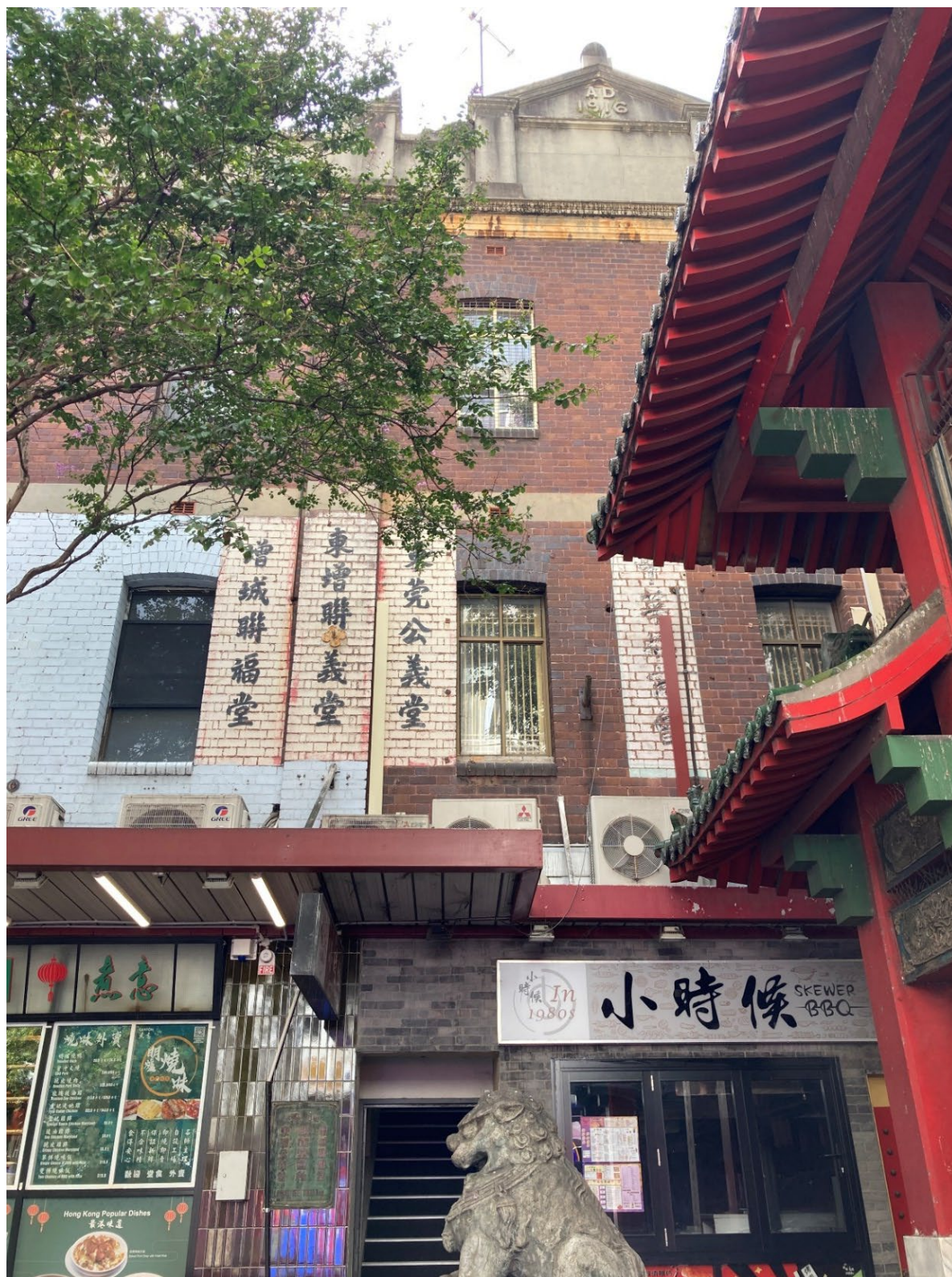
Figure 28. View of 52 Dixon Street. Source: HAA, 2024.
